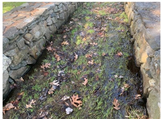
4 Brickyard Circle - 2 (Drainage Course)
