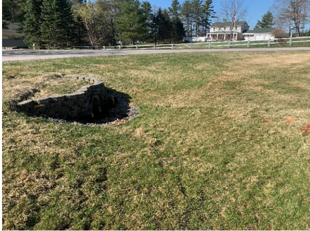
29 Gundalow - 1 (Drainage Area)
